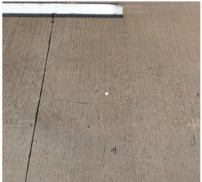
PHOTO 2 Description Typical unsealed cracks to Approach Slab.
