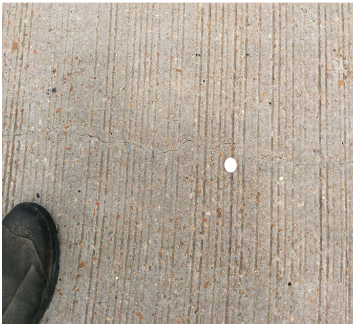
PHOTO 1 Description Typical unsealed deck cracks.
